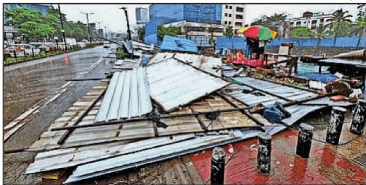
A makeshift wall collapsed in Baner on Thursday
